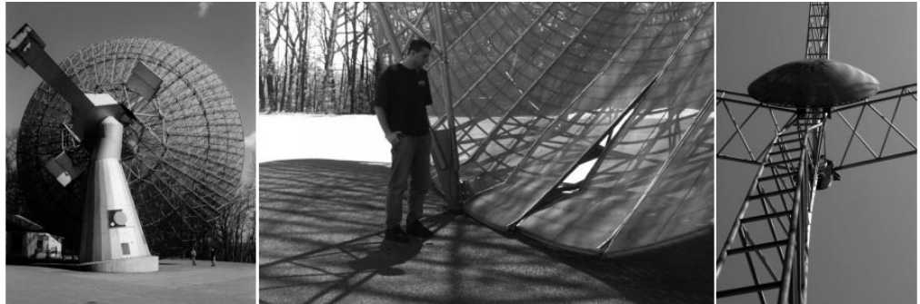
Figure 2. Fallen radiotelescope, damaged edge and secondary support.
