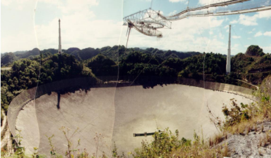
Figure 2.2: Showing the position of the catwalk above the Arecibo reflector. Looking closely, one can make out the dual helical feeds suspended from the catwalk. Shortly after this photograph was taken one feed was removed. Notice the substantial structure of the feed platform suspended above the dish and the line-feeds suspended from the azimuth arm. The ground-screen which surrounds the reflector was added in 1993 as part of the upgrade project.
