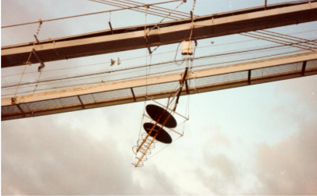
Figure 2.6: The dual helical feeds (before one was removed), suspended from the catwalk.
