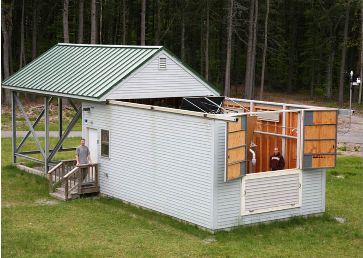
Figure 2.2: The wood-facade, steel truss observatory building has a roof that moves onto a steel support structure to the North along enclosed box tracks to expose the all-sky telescope. Barn doors open to the south for observations at low declinations. The Harvard clad object within is the author. Photo Credit: Paul Horowitz.
